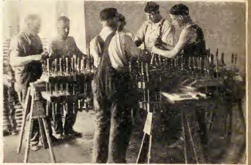
Glueing Propellers Blades
